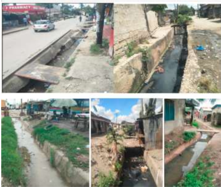
Figure 5.35: Informal Settlements Drainage Infrastructure
