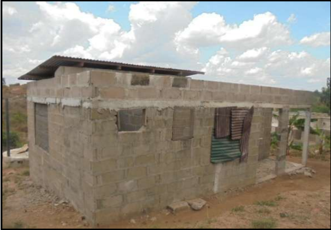
Plate 4. 13 Building construction at lintel level and occupied
