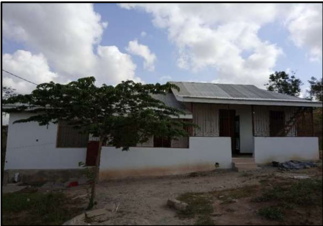
Plate 4. 14 Finished construction property and occupied
