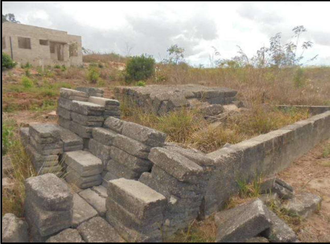
Plate 4. 11 Building construction stuck at foundation level
