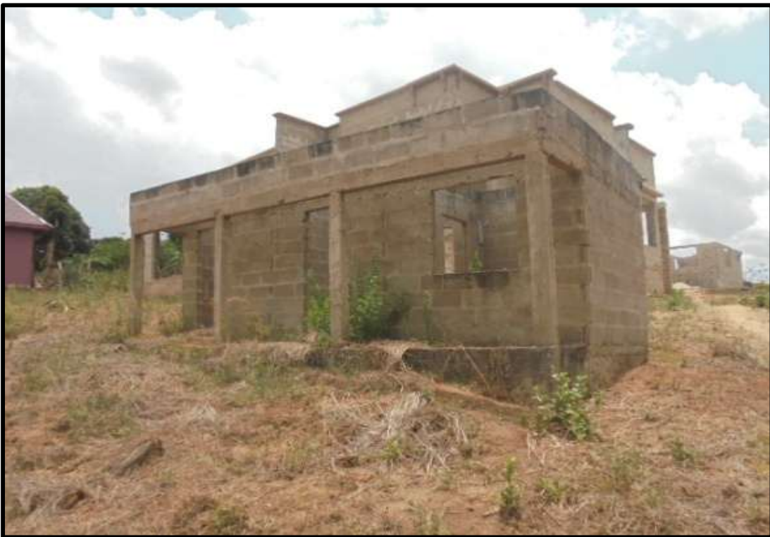
Plate 4. 12 Building construction at lintel level
