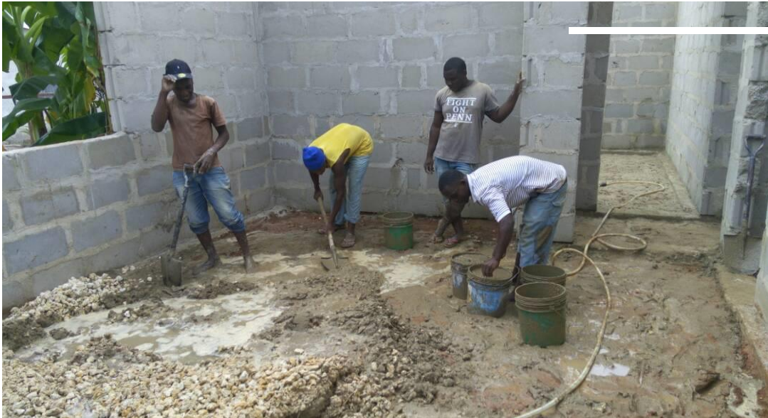
Plate 4.1: Unprotected Informal Construction Workers at Work.
