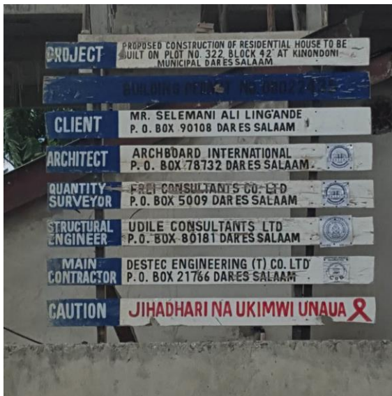
Figure 4.6: All stickers are pinned on the sign board during construction stage
