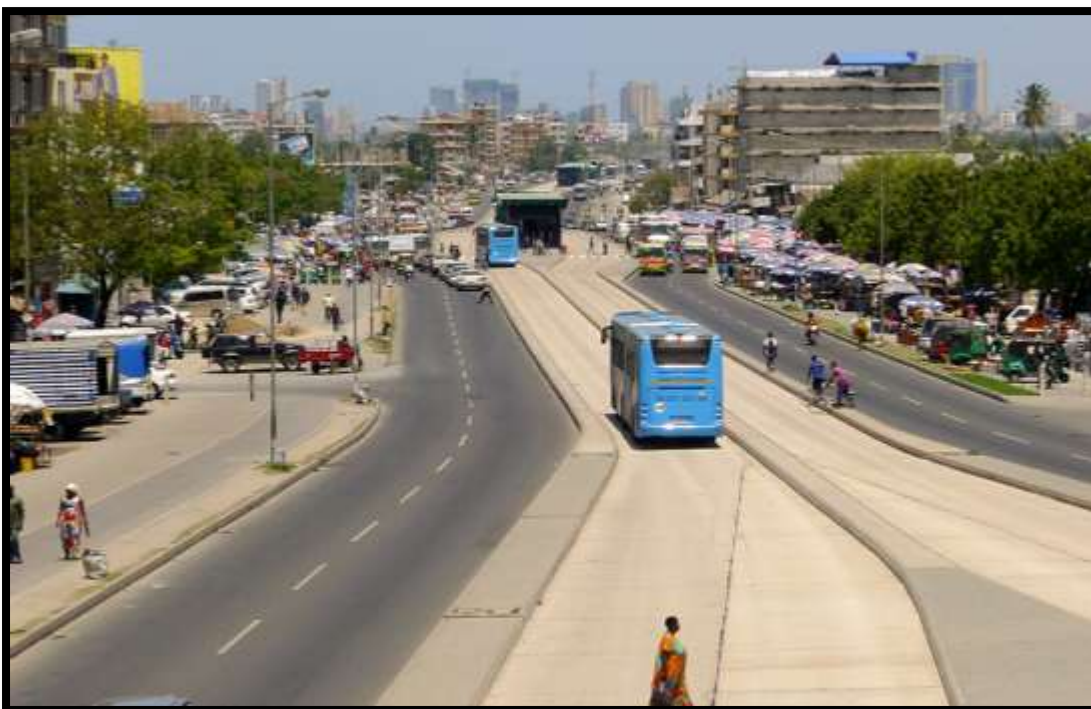
Figure 4.10: Pedestrians found crossing BRT road in non-zebra crossing area in Manzese.
