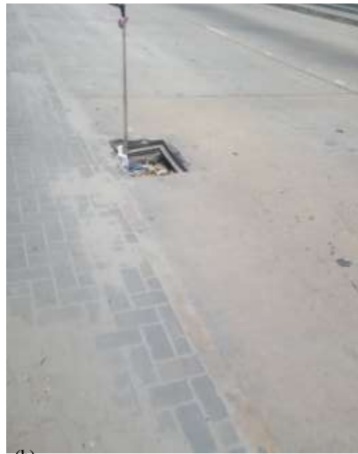
Figure 4.6: (a) and (b) Inspection chamber covered by vehicular tire in BRT road at DIT-Jiji bus station.
