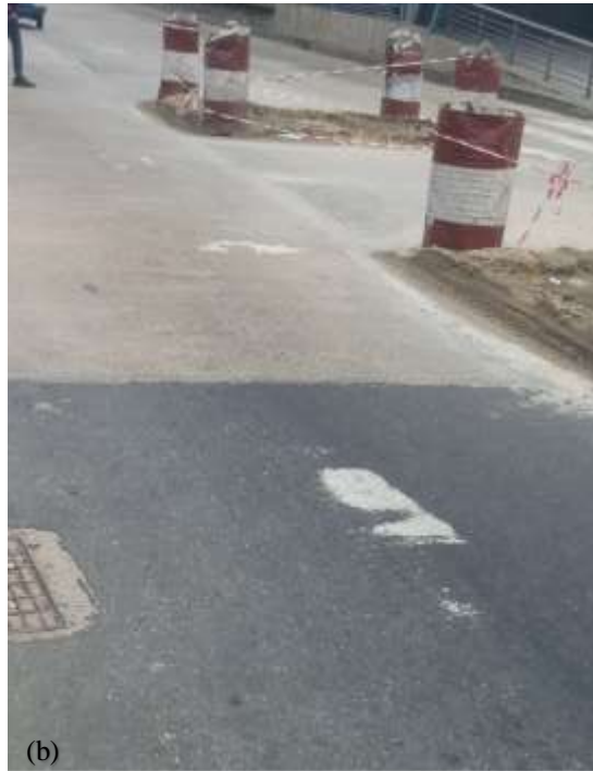
Figure 4.5: (a) Vegetation grows in pavement, (b) rehabilitation of road cracks at Kibo bust station.
