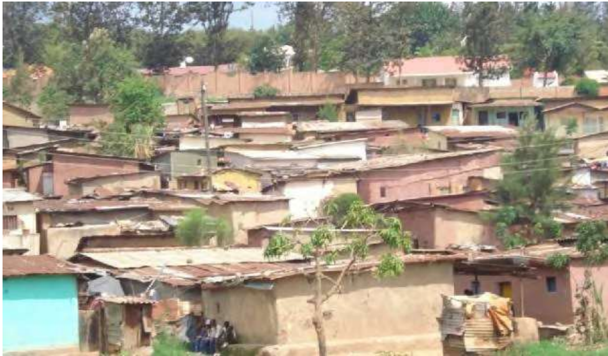
Plate 4 -1: Typical PAPs' former houses in Ubumwe prior to relocation
